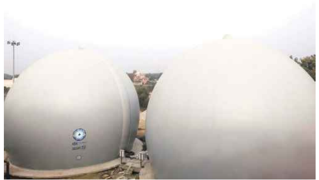
140 MLD STP at Dinapur, Uttar Pradesh
